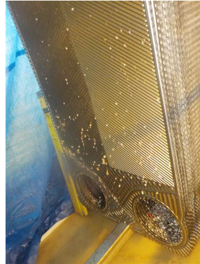
Forward engine cooler No biological or mineral fouling
