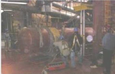
With air caster, just a few people are needed to move a 50 ton unit.
