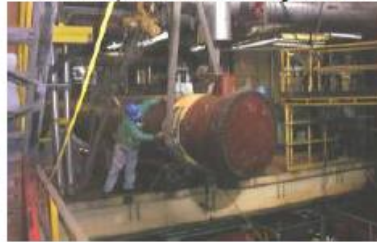
Heater is in position for the crane to grab an end
