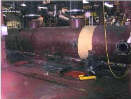
AeroGo air casters are inserted under the load prior to moving.
