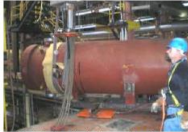
Heater is in position for the crane to grab an end
